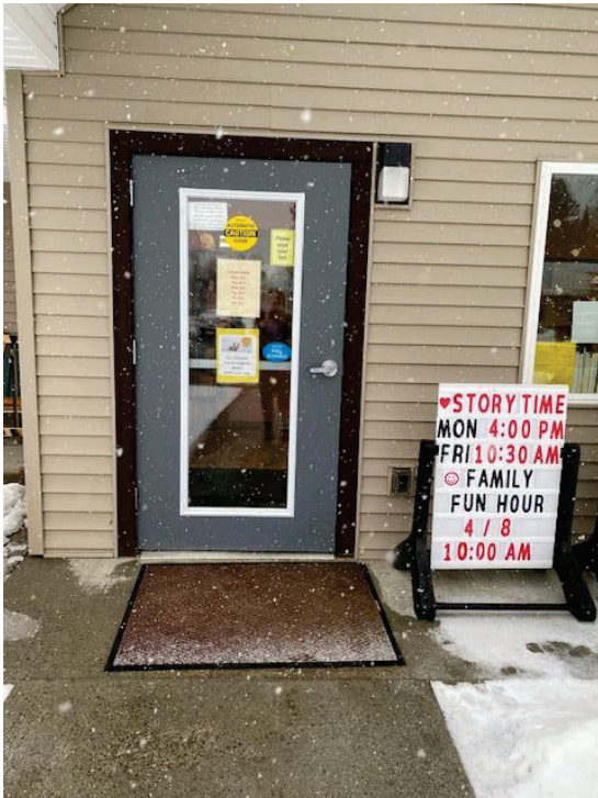
Photo 1: Current front door, straight on from front walkway, facing south.
