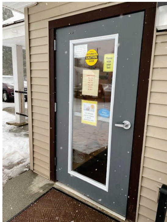
Photo 2: Front door looking toward east parking lot.
