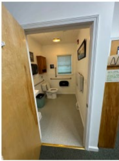
Existing Main Level Bathroom
