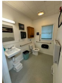
Existing Main Level Bathroom
