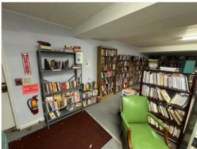
Basement area where new lower level bathroom will be located. There is no bathroom on this level currently.
