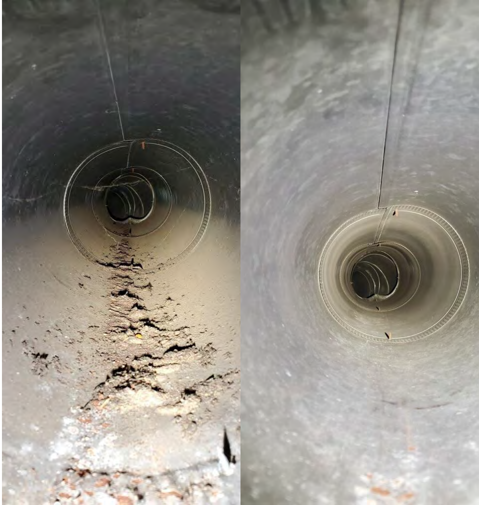
BOLTON FREE LIBRARY DUCTWORK #1 BEFORE & AFTER PHOTOS FEBRUARY 2024
