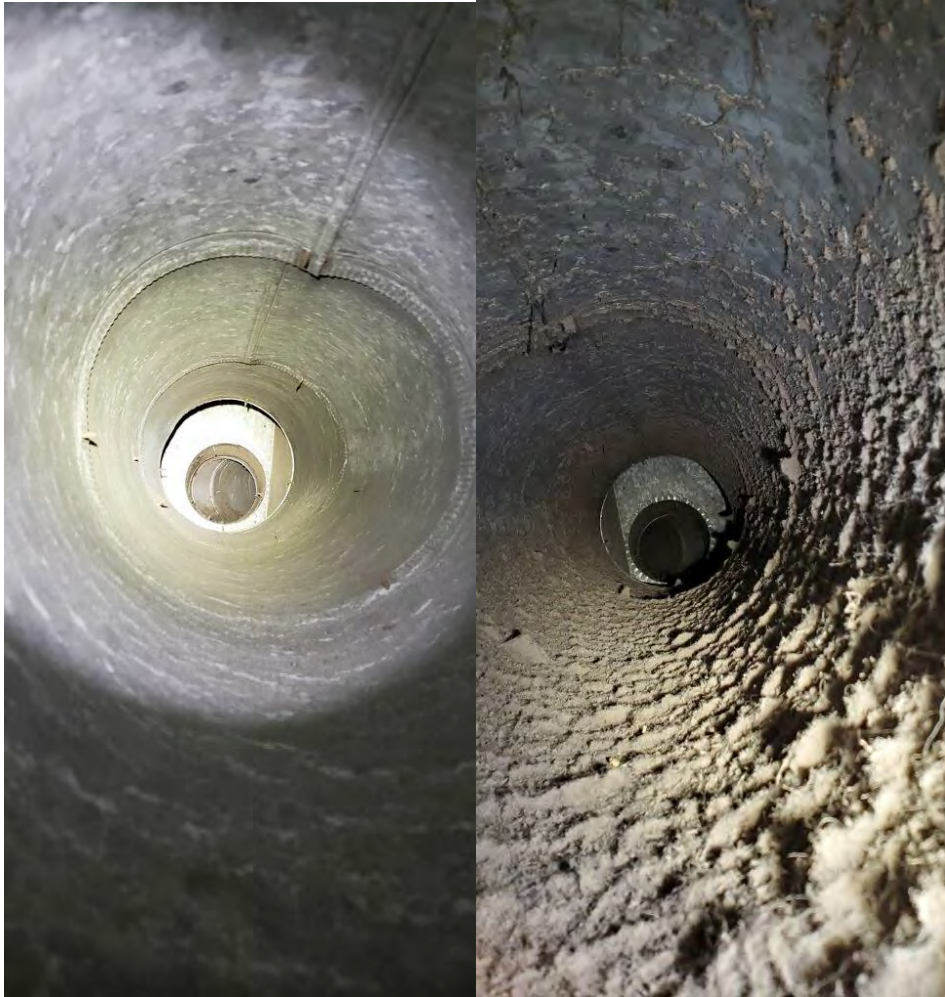
BOLTON FREE LIBRARY DUCTWORK #2 BEFORE & AFTER PHOTOS FEBRUARY 2024
