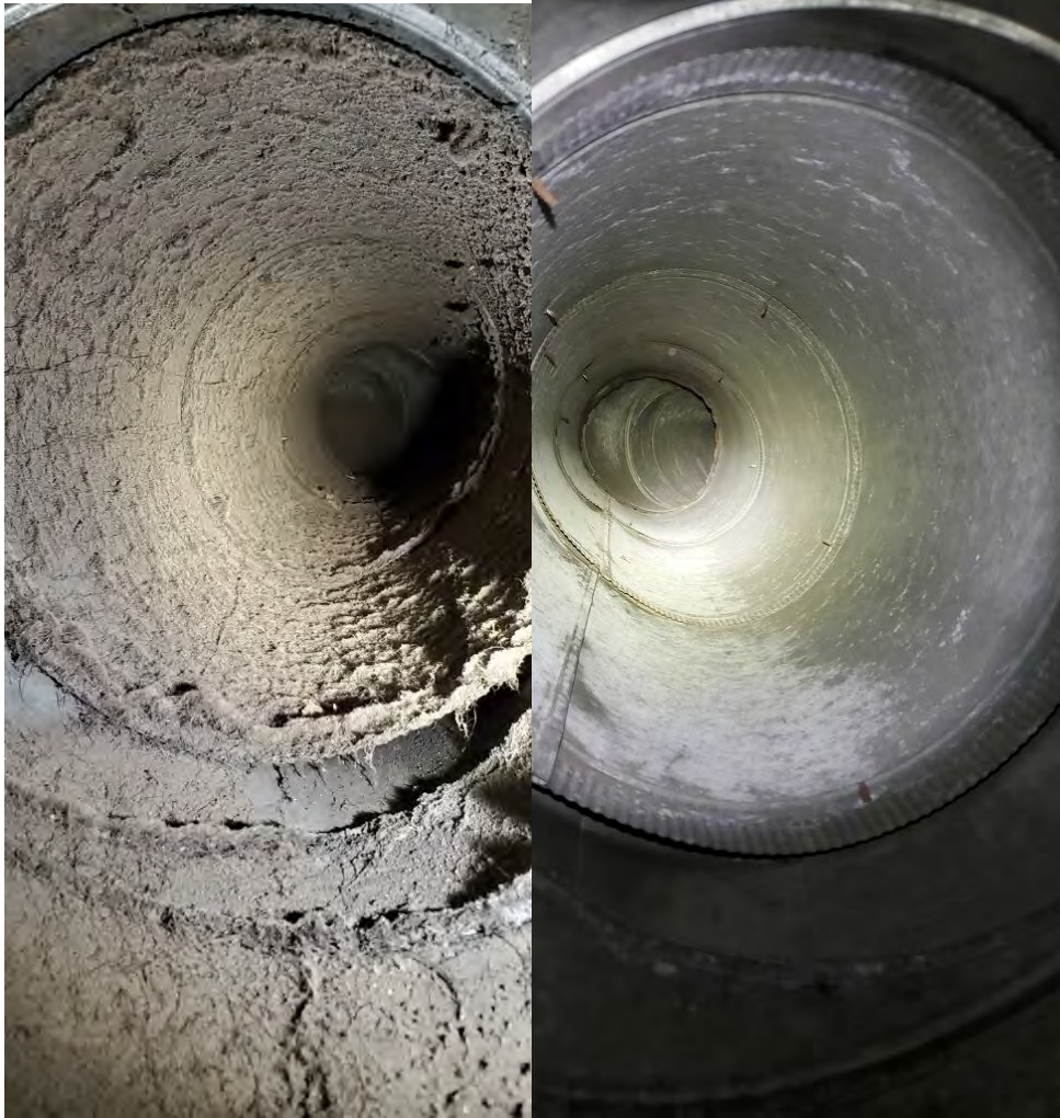
BOLTON FREE LIBRARY DUCTWORK #3 BEFORE & AFTER PHOTOS FEBRUARY 2024
